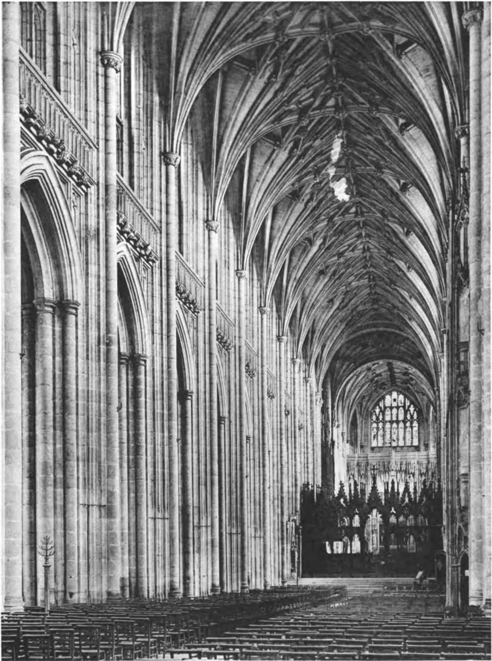
WINCHESTER CATHEDRAL, NAVE FROM S.W.
