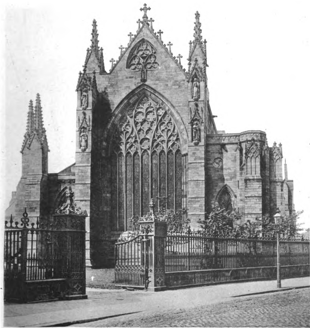
CARLISLE CATHEDRAL, EAST FRONT.
