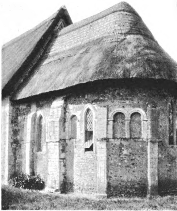
Hales, Exterior of Apse.
