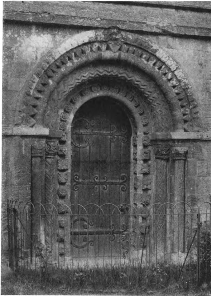
Iffley South Doorway.
